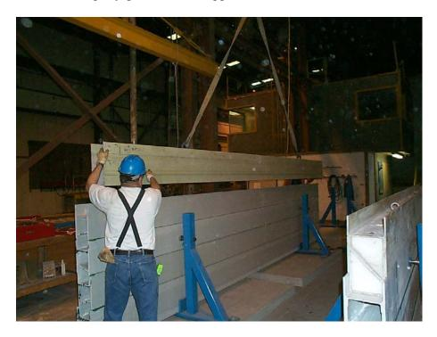
Figure 11. Bonding Deck Tubes to Make Panels for the Bridge Installation.
